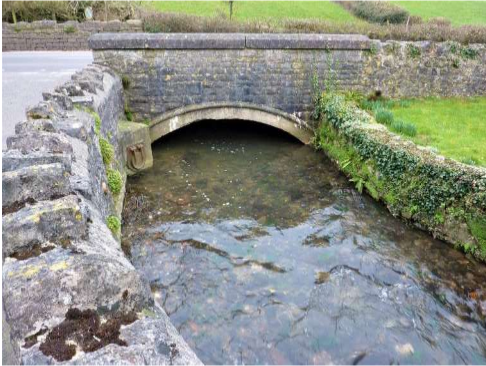
Figure 14: The River Sheppey downstream of Ham Mill
