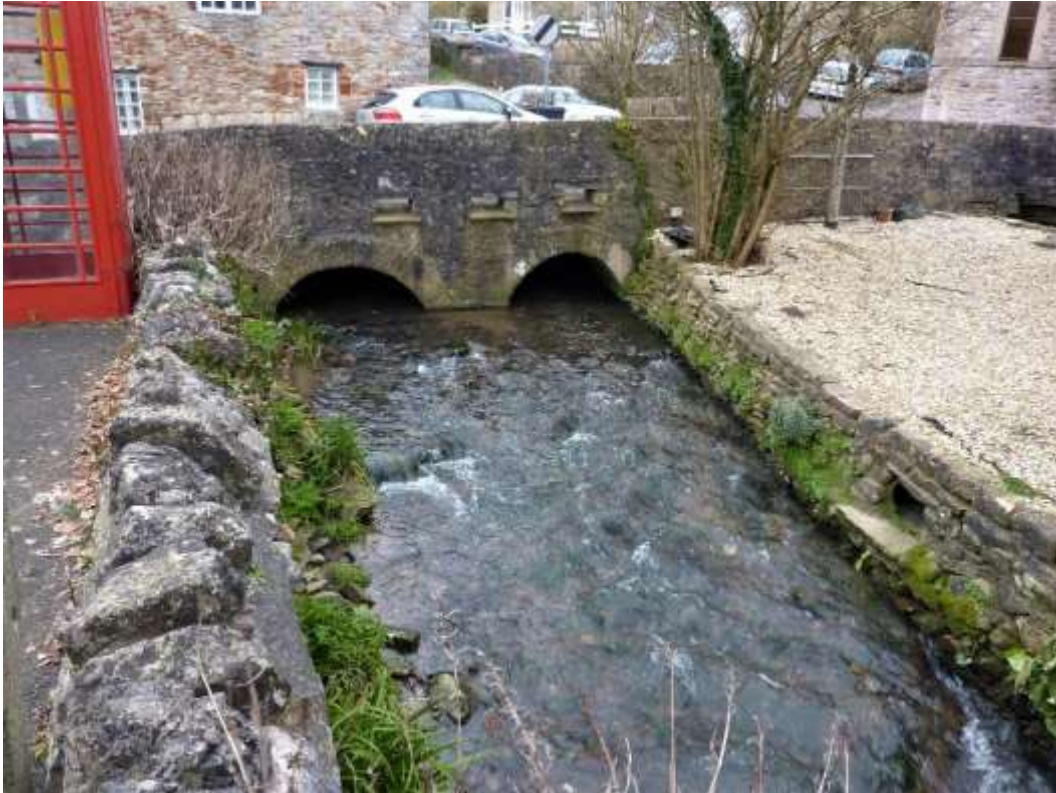
Figure 12: At Old Street Lane bridge, small marginal berms could be formalised, with small but significant habitat and visual benefits. In this area and further downstream, small perturbation boulders could also be added to increase habitat diversity
