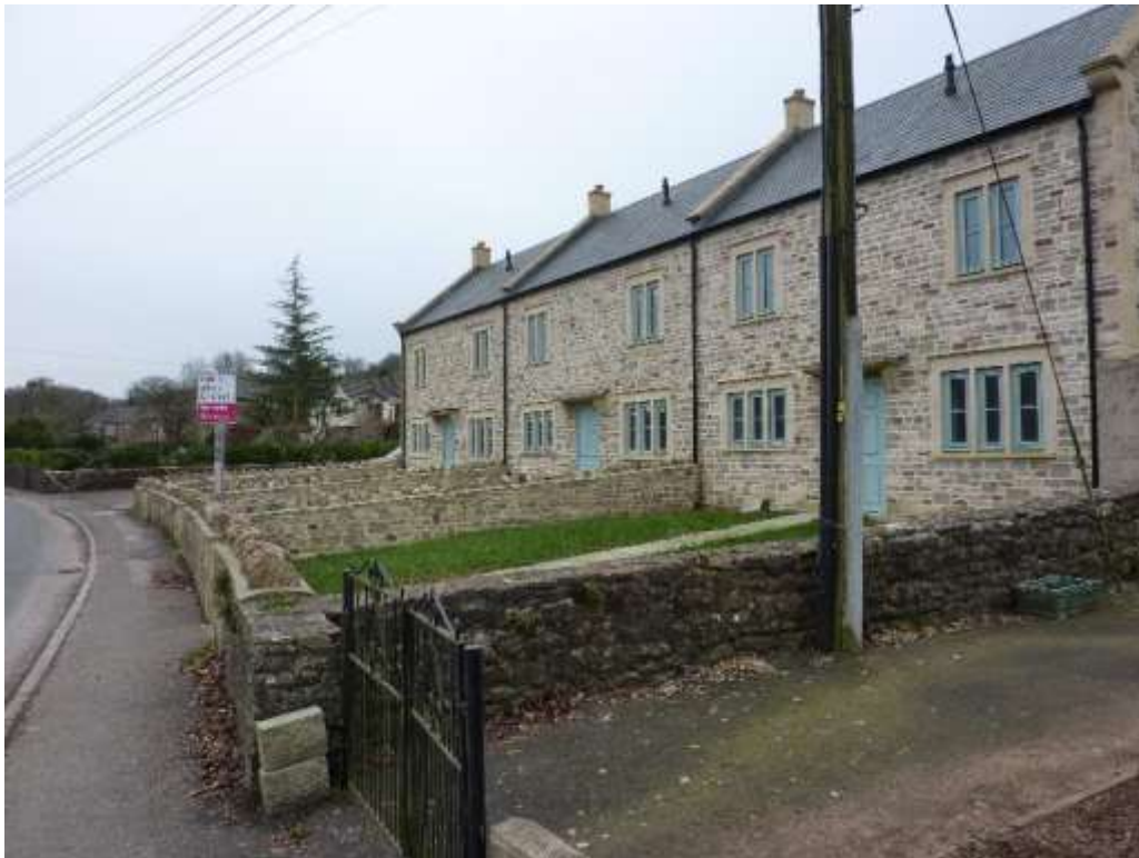
Figure 13: A recent housing development along the A371, with the River Sheppey disappointingly still culverted under its front gardens – a major missed opportunity to reduce flood risk and increase the aesthetics of the village
