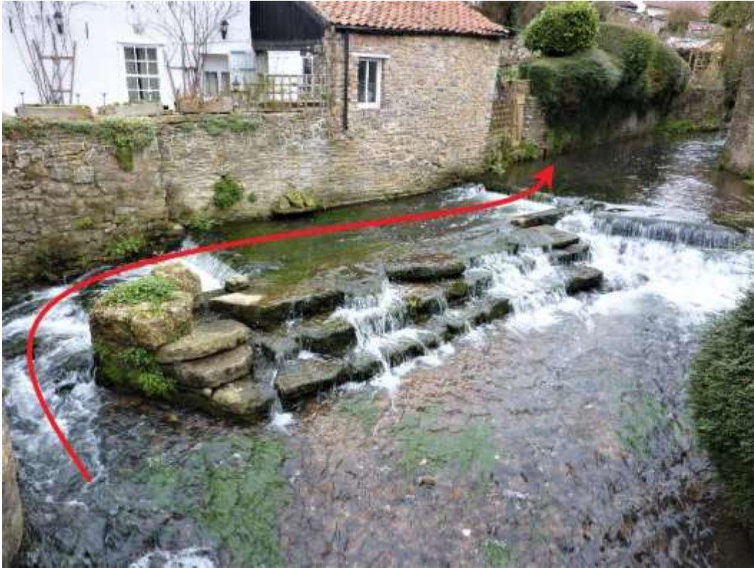
Figure 9: A complex system of weirs beside the village school, with an arrow showing a potential fish passage easement route after removing modern weir sills
