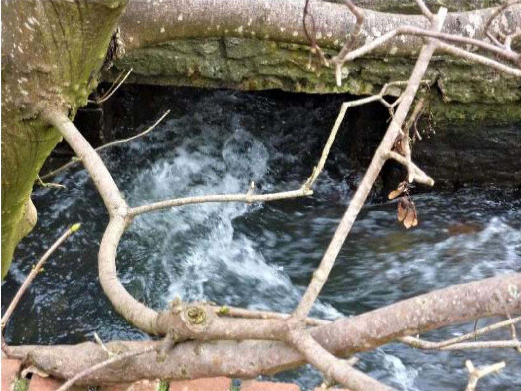
Figure 11: A dog-leg culvert, with integrated weir(s), under Old Street Lane
