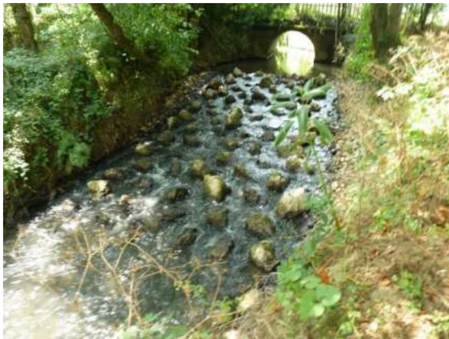
Figure 18: A rock ramp is an effective fish passage solution when a culvert cannot be modified with baffles or other easements, and a step up into it may need to be 'drowned out'. This example uses a series of erratic perturbation boulders to baffle the flow and ease fish passage.
