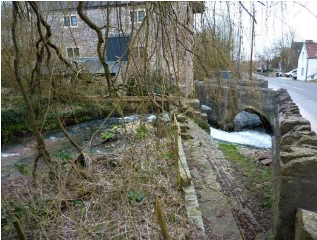
Figure 6: An impassable weir between Duncart Lane and Back Lane
