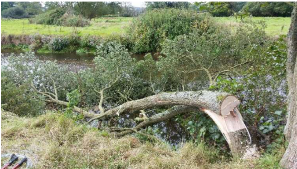
Figure 16: To reduce overshading and increase habitat, bankside trees can be hinged into the edge of a river so that they can continue to grow (depending on species) and provide low-level cover for fish, insects and birds. For extra security, the branches can be staked, or the trunk can be cabled back to the stump.
