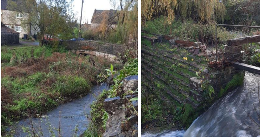
Figure 22: Upstream of Duncart Lane Bridge and Old Mill weir
