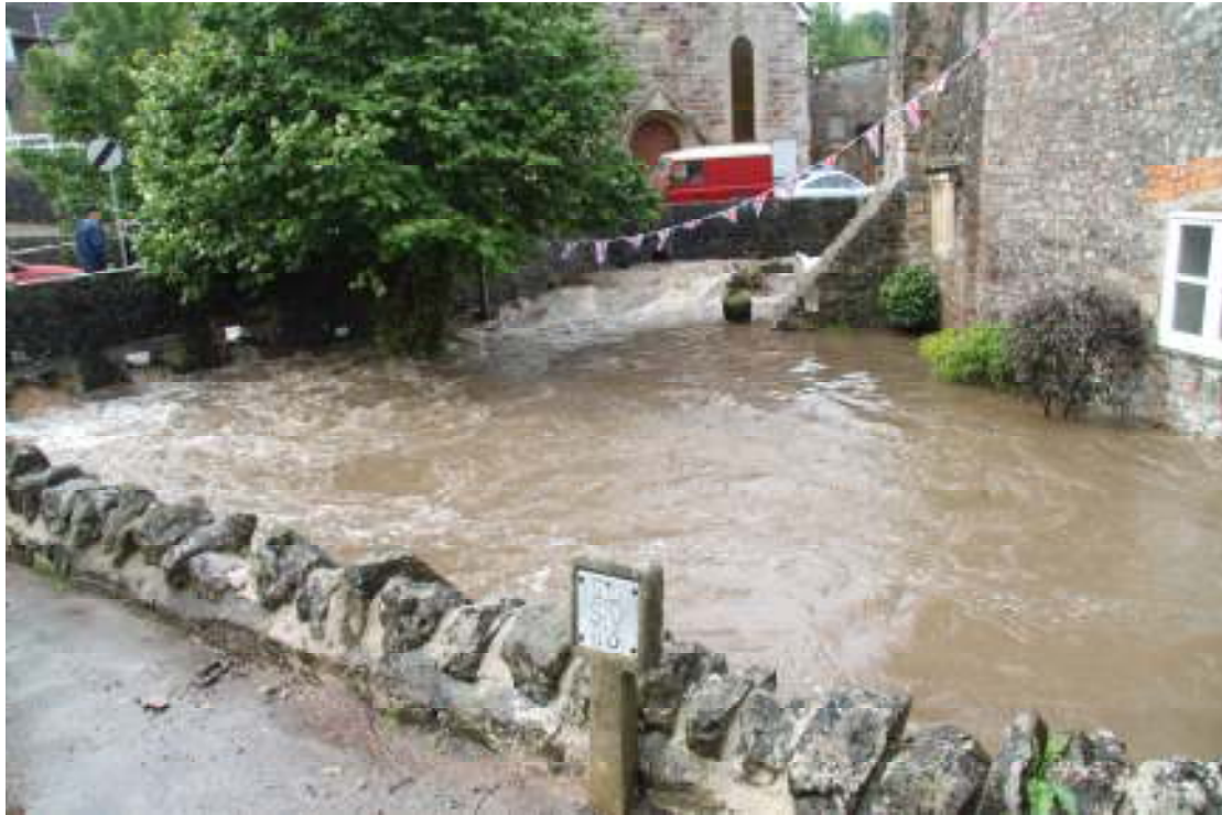
Photograph 5 - Manor House at peak river levels
