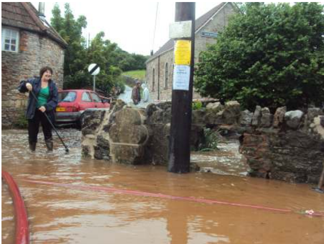
Photograph 4 - Long Street showing opening through wall
