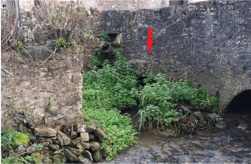
Figure 14 - Jack's Bridge showing the culvert adjacent to A371 Long Street blocked with vegetation
