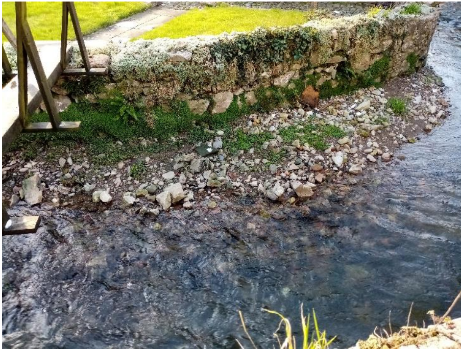
Figure 18 - River Sheppey inside bend deposition (A371 Long Street and Fayre Way junction)
