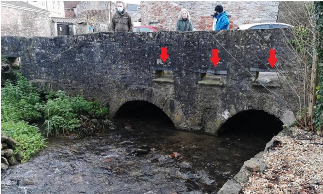
Figure 15 - Jack's Bridge downstream parapet with three spillways
