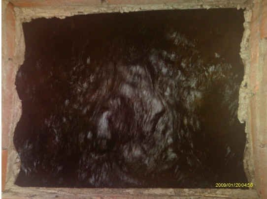
Site Photos - SMH1 Chamber
